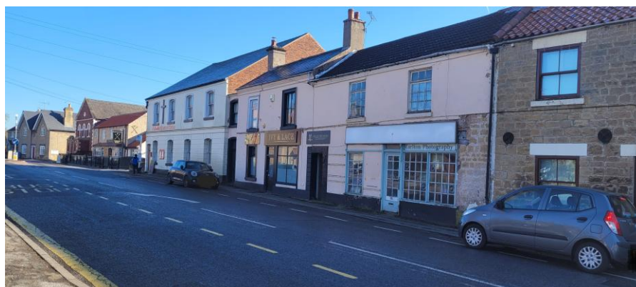
Shops – High Road Local Centre
