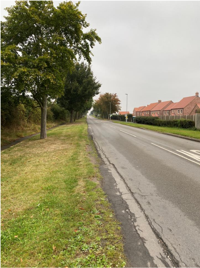
KV20: Looking north along Mattersey Road wide grass verges are retained as part of new development – demonstrates contribution street trees and wide verges make for soft transition to countryside.
