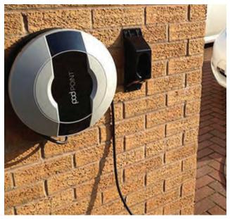
Figure 94: Home electric vehicle charging point.
