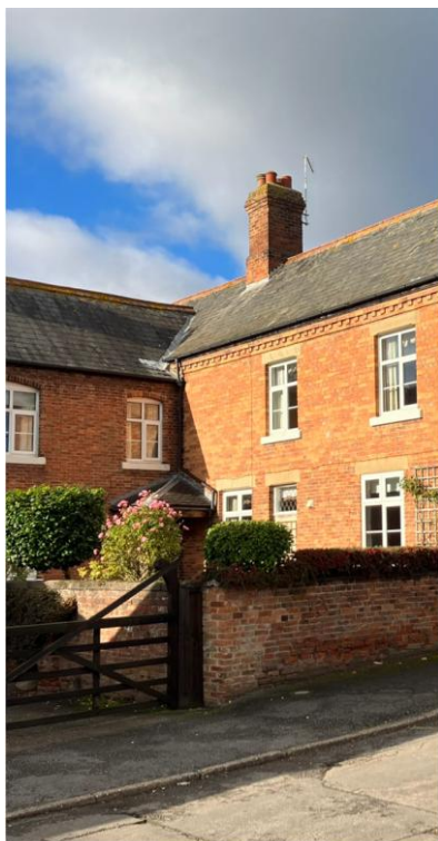
Photo 1: The vernacular and agrarian nature of Elkesley's historic building stock means that many existing sites have traditional agricultural 'courtyards'
