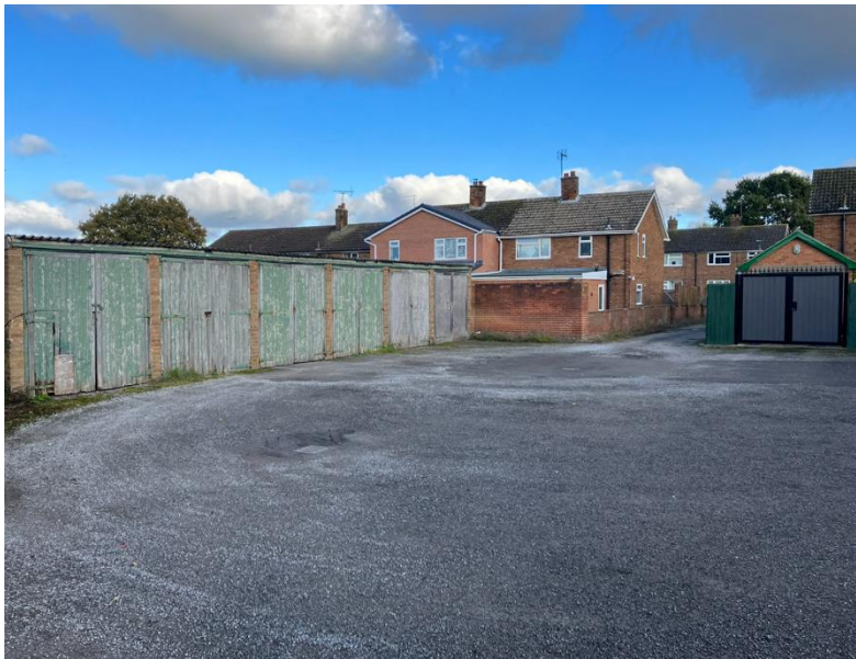
Photo 15: Site 2 Garage site off Lawnwood Avenue
