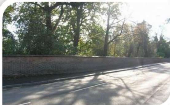
Pictured above: Boundary wall next to Hospital Road and Rectory Road.
