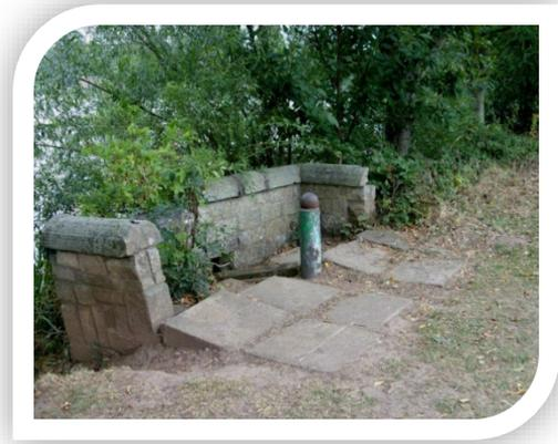
The weir between the Upper and Lower Lakes which has been rebuilt sympathetically in the 1980's to provide safe access for the lakeside circular walk. The main dam of the Lower Lake and sluice have also been substantially rebuilt/strengthened in the 1970's to ensure the lakes meet the requirements of the 1975 Reservoirs Act. This followed a number of dam failures and leakages earlier in the 20<sup>th</sup> Century.
