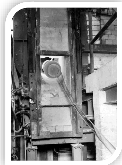
Pictured above: CWS Glass Works, Sandy Lane, Worksop. View of molten glass being squeezed into a long strip. Taken about 1940
