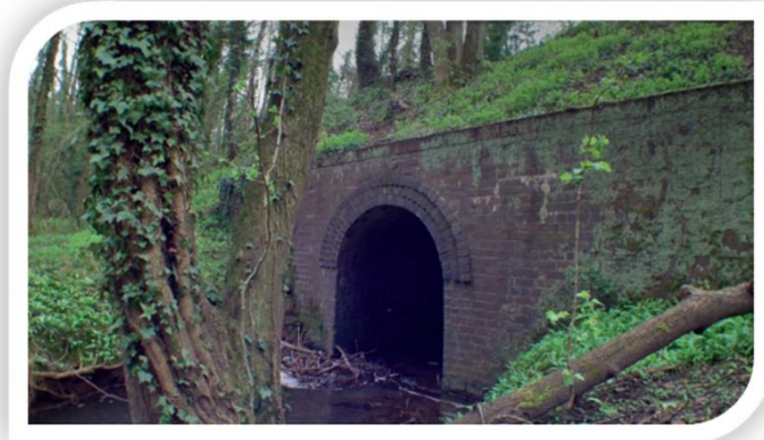
Pictured above: The culvert near the Costhorpe Plantation.
