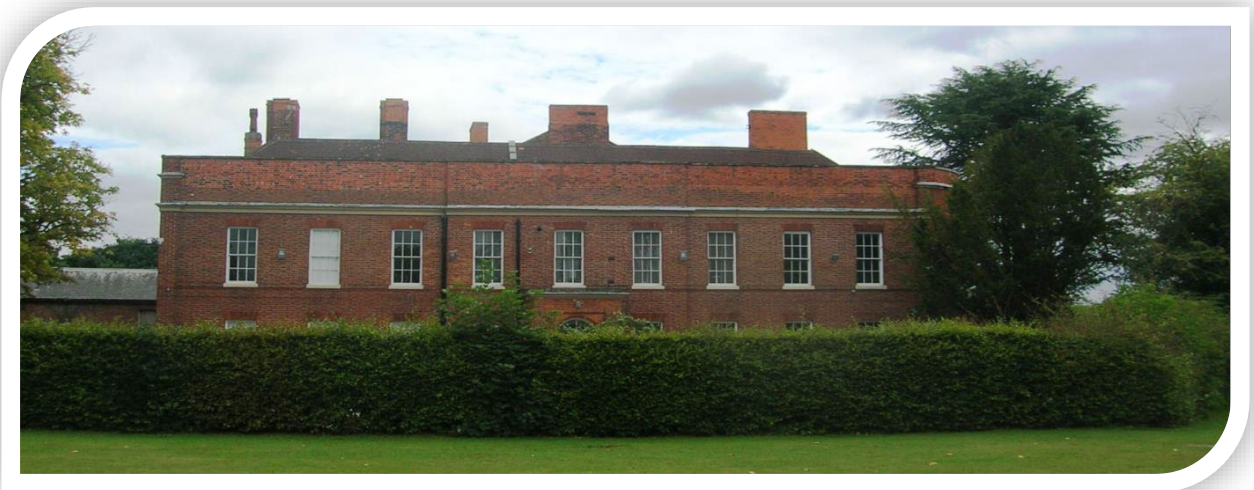
Above: Main façade of West Retford Hall
