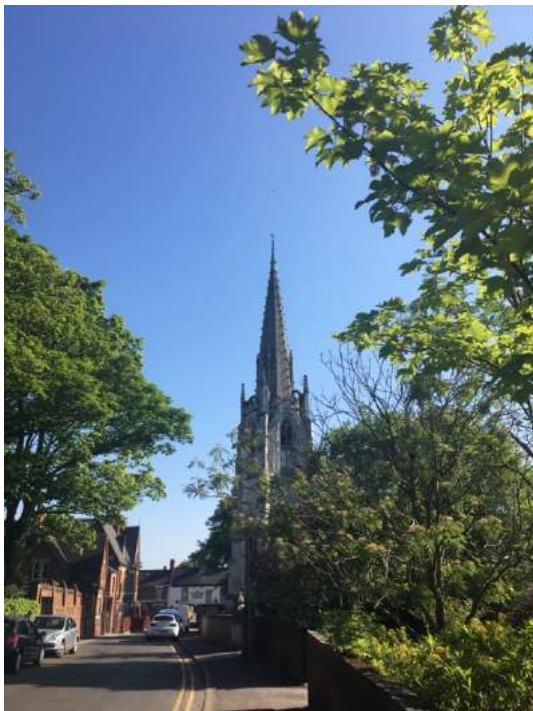
KV 2 Looking north east along Rectory Road to St Michael the Archangel – a key landmark building Grade 2*
