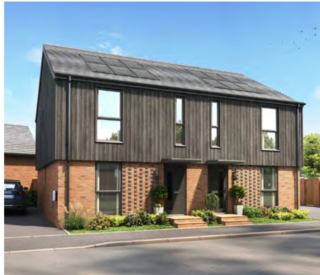
Figure 74: Carbon negative affordable homes in Derbyshire.
