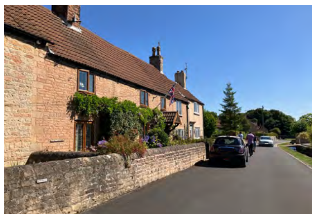
Figure 69: Properties on Queens Walk in the Conservation Area
