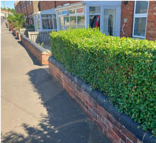
Figure 64: Boundary materials should aim to reflect the materials and colour of the related property and the character area in which it resides. The characteristics of each character areas are set out in chapter 03.
