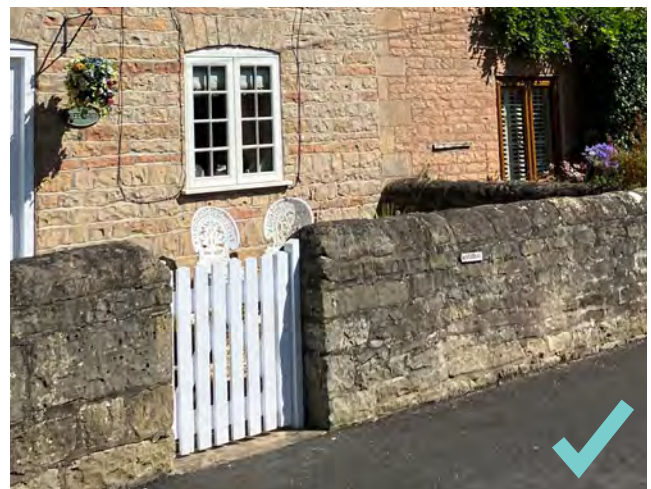
Figure 73: Stone boundary walls delineating between public and private space
