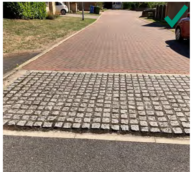
Figure 63: Change in surface materials and colours delineating between primary, secondary and tertiary streets.
