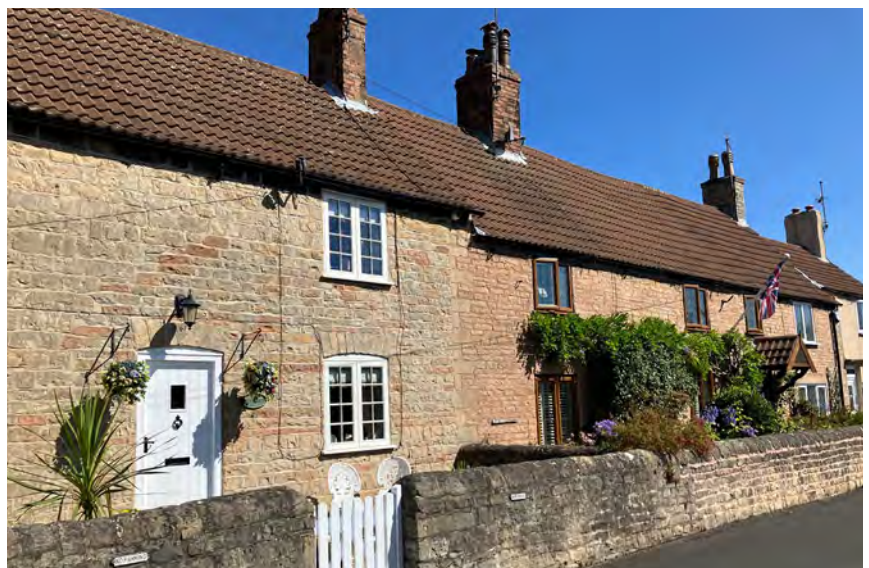
Figure 20: Terraces fronting the Green, Queens Walk
