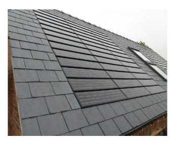
Figure 70: Integrated solar panels on slate roof.
