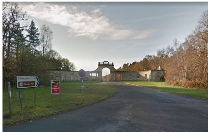
Figure 5.1: Entrance gate to Lime Tree Avenue, as viewed from A614 40
