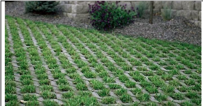
Example of geopaving, flowering perennials could also be planted to provide higher biodiversity value.
