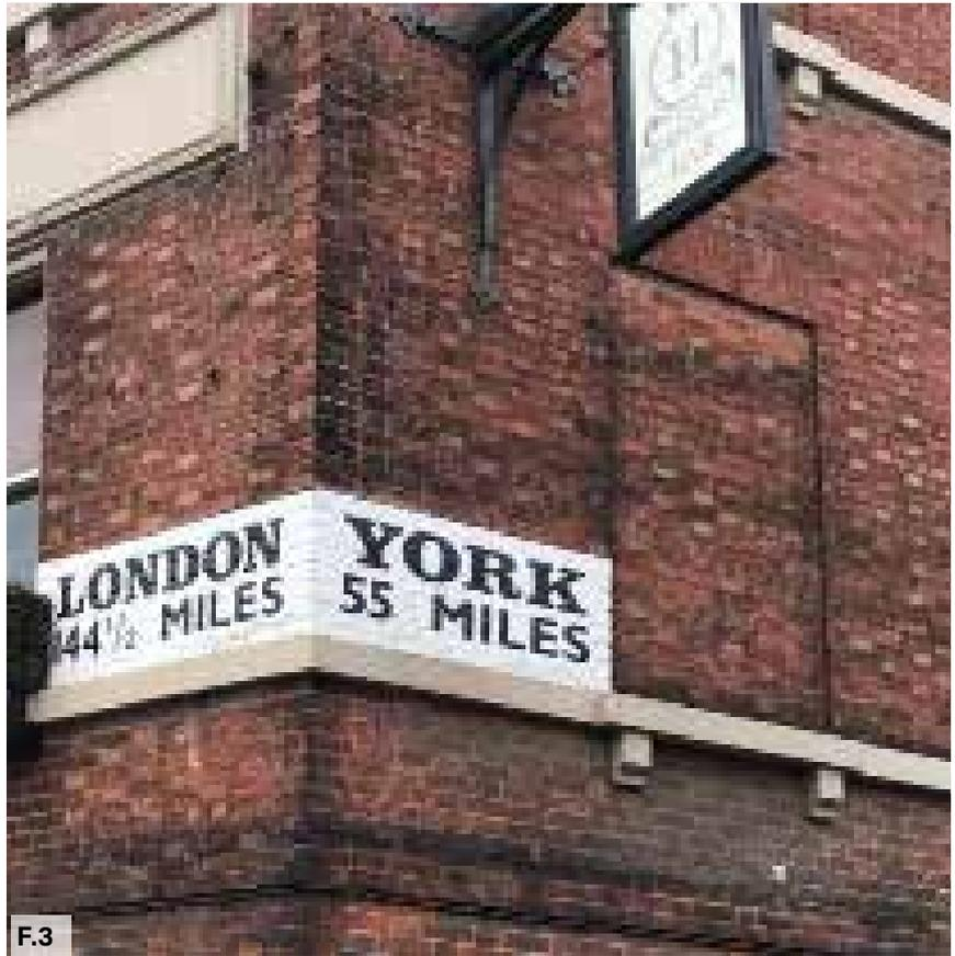
**Figure 02:** Contrasting coloured Flemish bond brick elevation on Market Square
