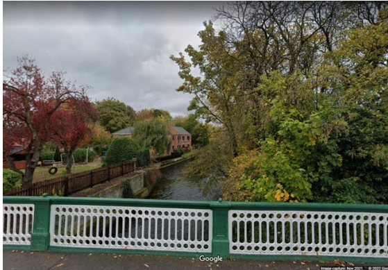
KV 3a Bridgegate looking north east along the River Idle – a main corridor for wildlife with mature trees that planting – a green ribbon that runs north south and is a backdrop of the urban area
