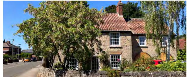
Figure 42: Stone Cottage on the junction of Main Road and Queens Walk
