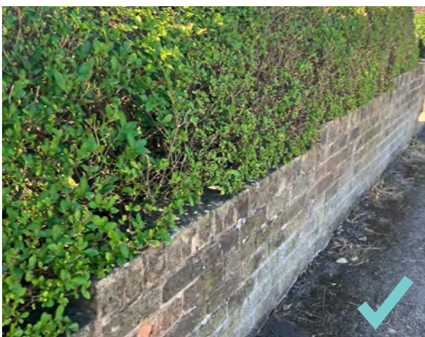
Figure 72: Boundary walls supported by hedgerow delineating between public and private space
