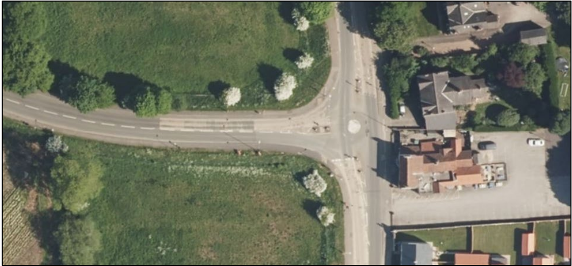
Image 3 – (J14) A638 London Road / Whitehouses Road Mini-Roundabout Junction
