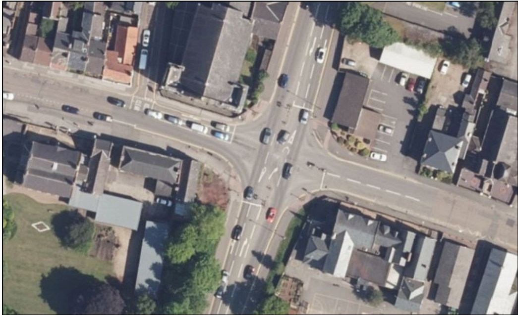
Image 5 – A638 Arlington Way / Grove Street Junction (J11)
