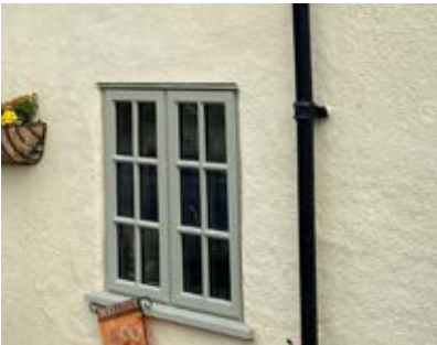
Casement window with timber framing
