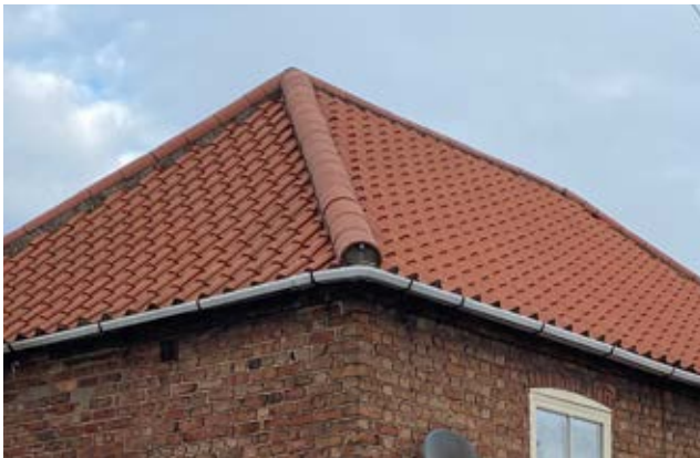
Misterton's traditional roof material. Red pantiles are typical of the regions historic roofscapes.
