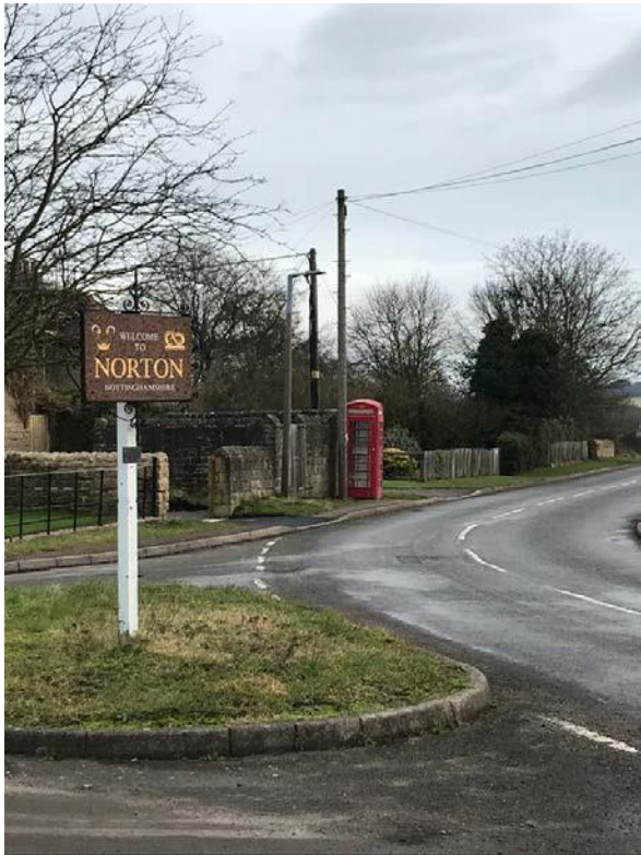
View number 4 junction of Main Street and Lime Street Avenue looking west within the Conservation Area, captures the traditional heritage features, boundary treatment, use of local stone.
