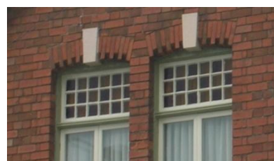
Figure 3.16: Transom windows with coloured glass at 23 Blyth Road.
