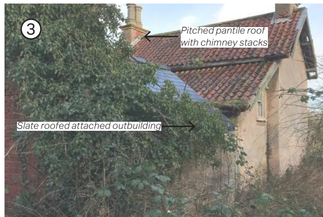
3. Rear of Eddison's Cottage and outbuilding, Norton
