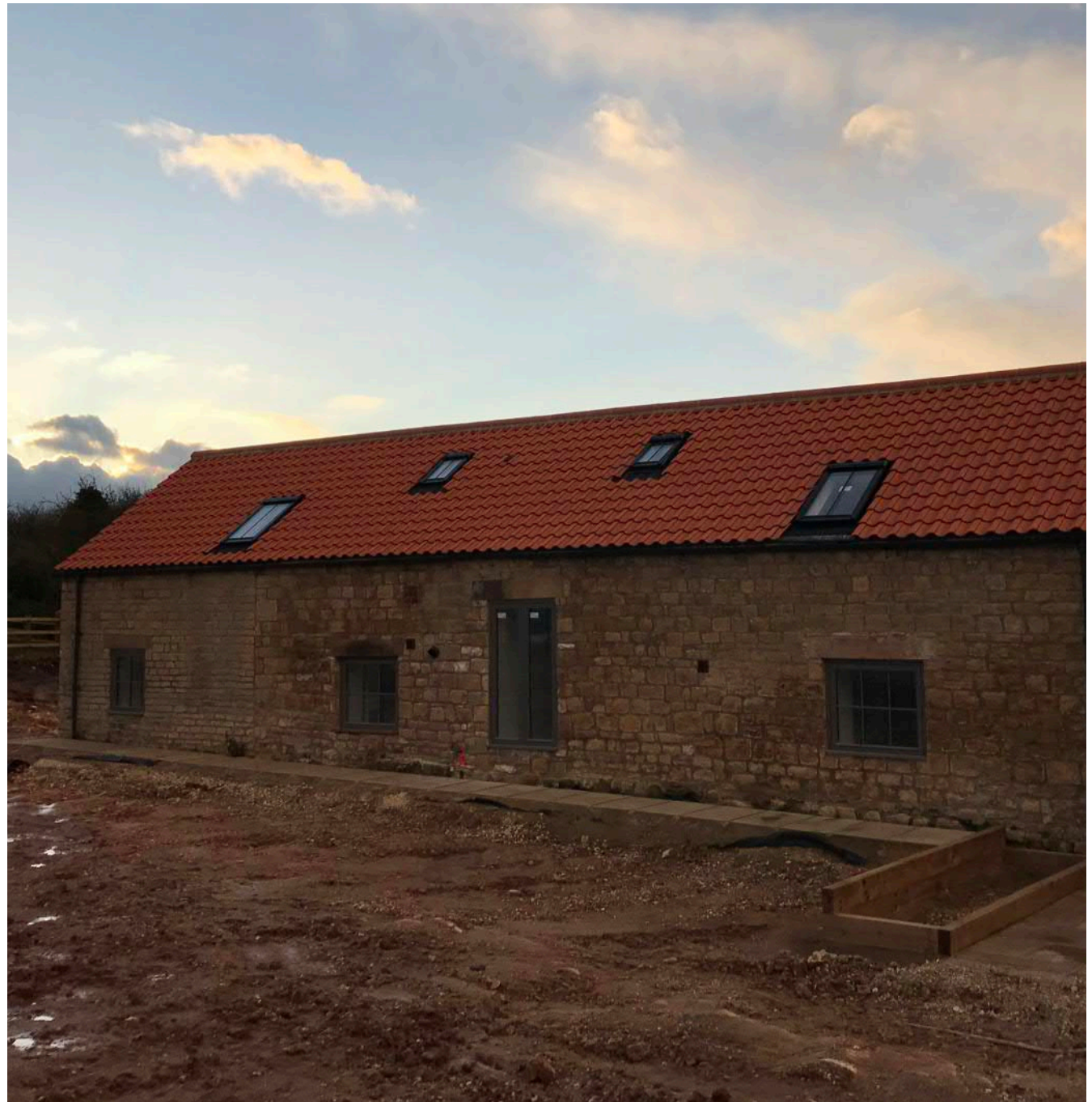
Farm buildings being converted to residential use in Belph (just outside of the Neighbourhood Plan area)
