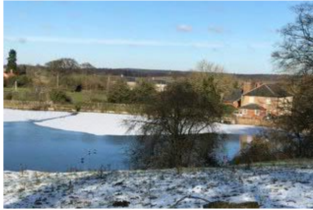
5. View of Cuckney Dam
