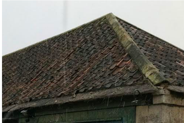
Hipped roof form
