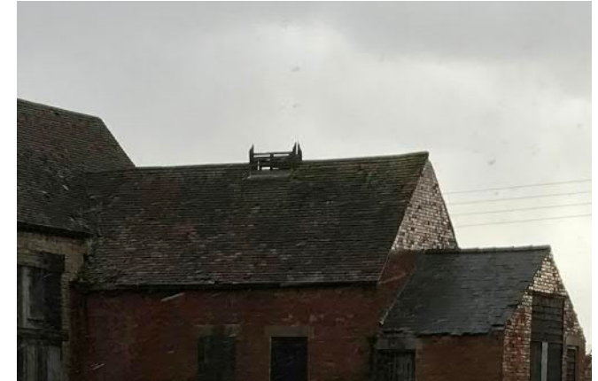
Stepped gable roof forms
