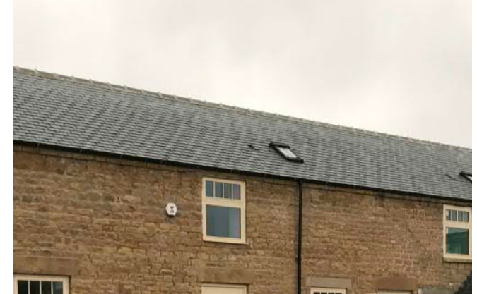
A former asbestos cement roof re-covered with slate
