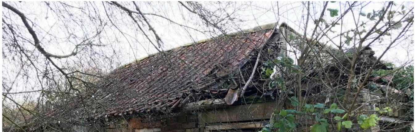
A dilapidated hipped roof form
