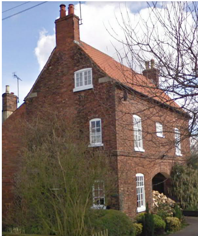
2.5 storey dwelling using roof space, Norton
