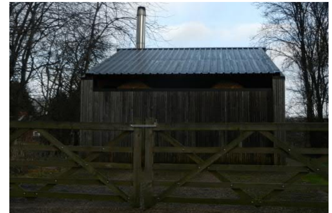
Wood chip biodigester, Norton
