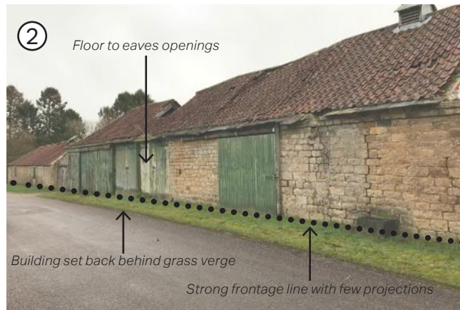
2. Vacant farmstead buildings, Holbeck
