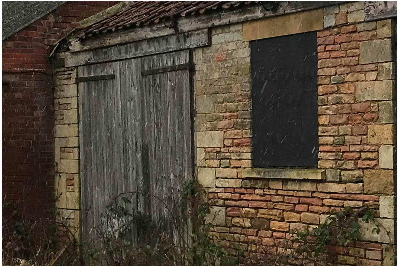
Boarded up openings can be reinstated and details such as stone sills, lintels and quoined corner detailing should be preserved
