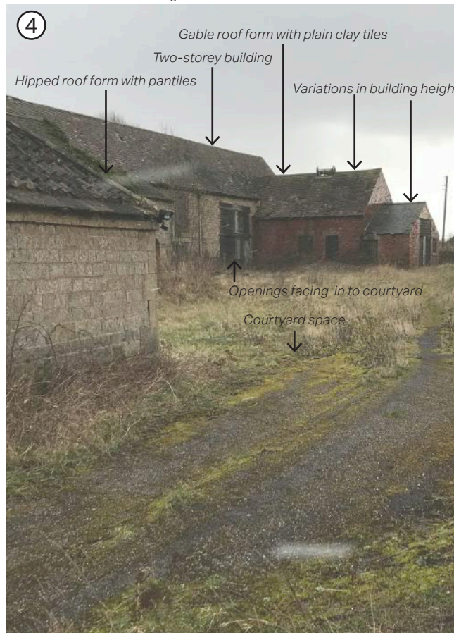
4. Vacant farmstead buildings, Holbeck
