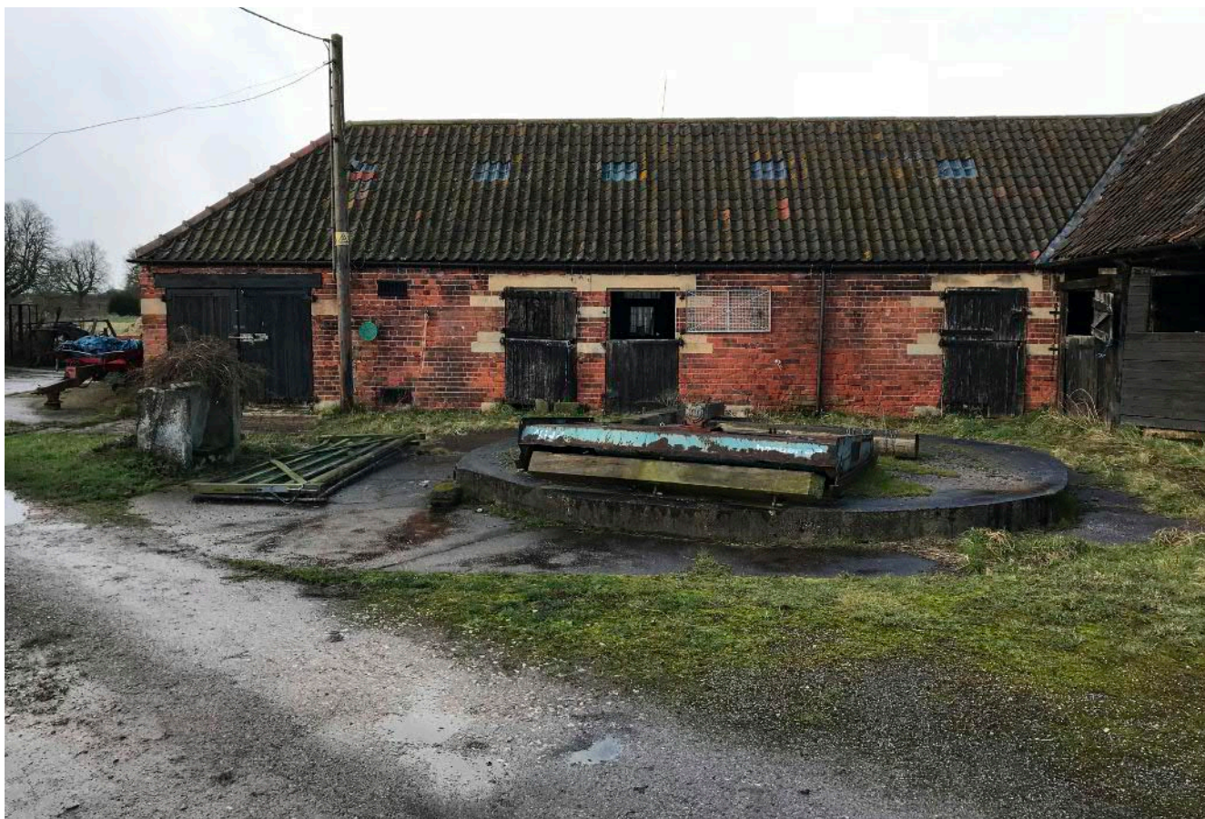
An L Shaped building with the principal elevation facing south in to a courtyard space
