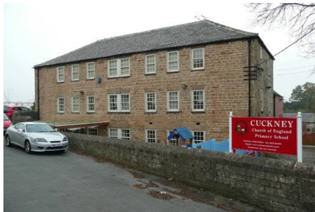
3 storey former mill building, Cuckney
