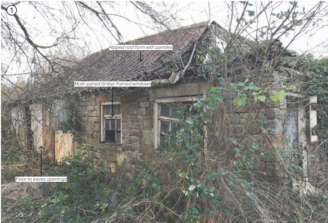
1. Dilapidated outbuildings, Norton
