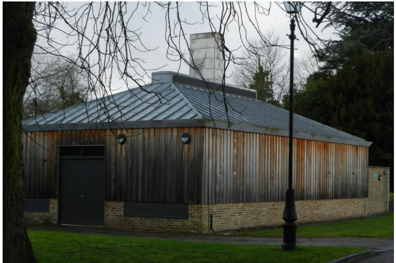
Welbeck's 800kw Biomass boiler
