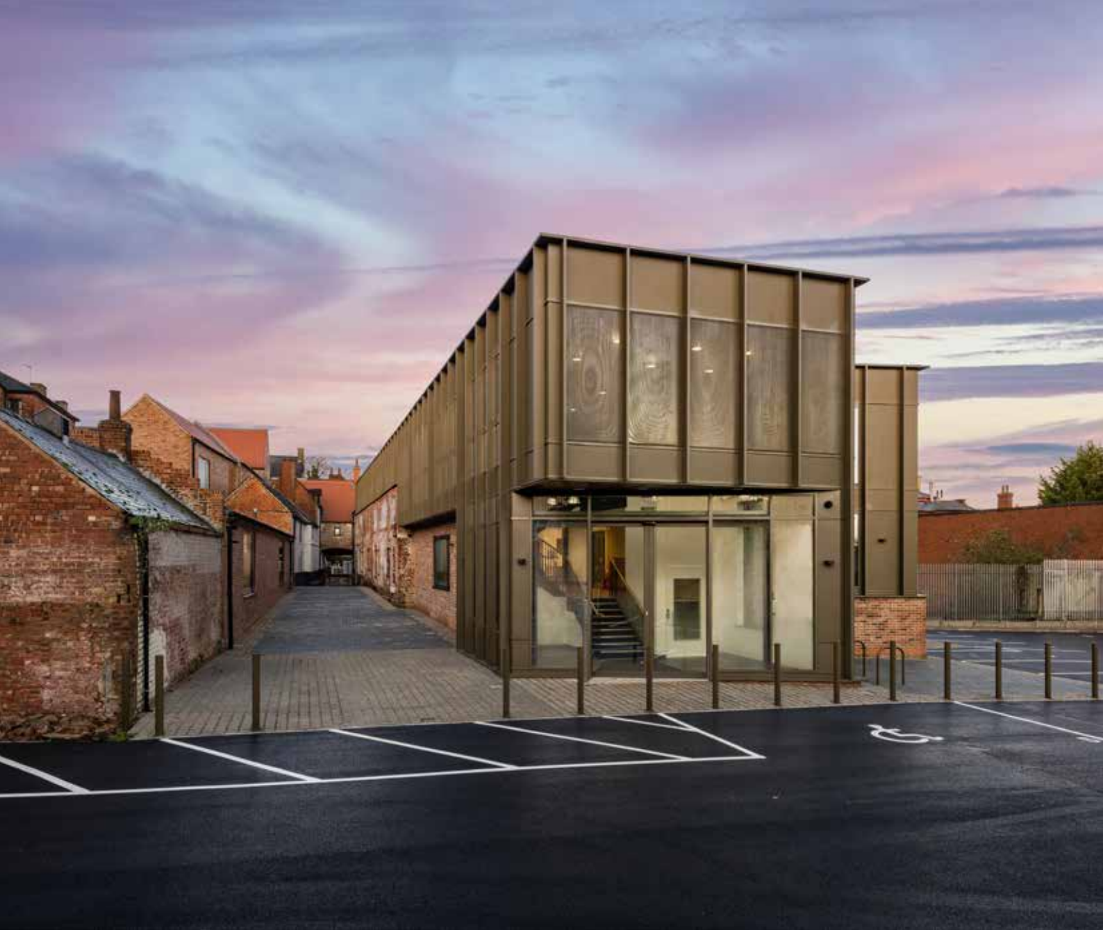
Middletons Yard, Worksop
