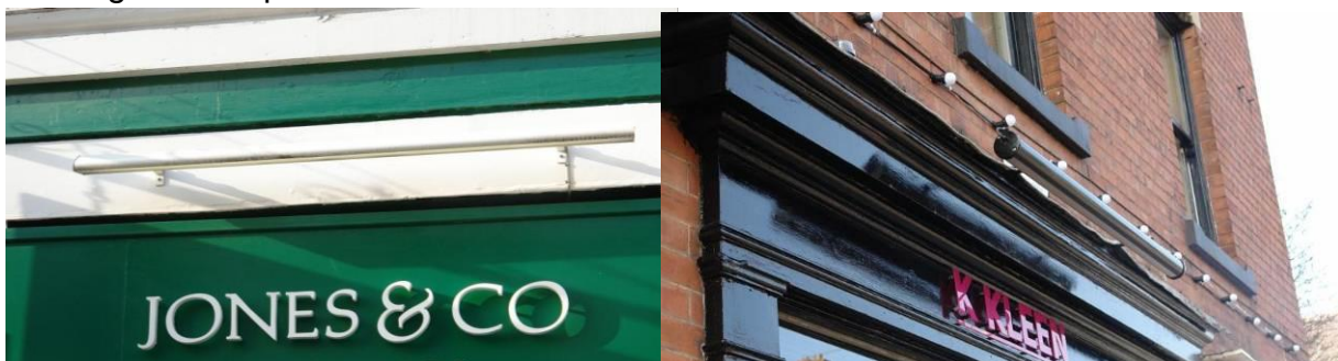
Figure 47. Fluorescent tube lights coloured to match the fascia.
