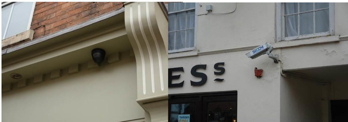
Figure 59. Left; discrete dome camera on underside of modern cornice. Right; unsightly overly large camera focused on entrance doors.
