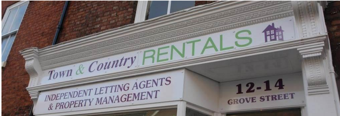
Figure 30. Pre-formed signage attached to fascia with screws and visible studs.
