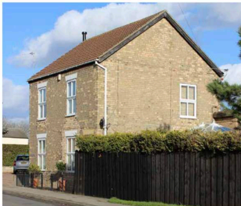
Figure 45: SW.02 - The Walkeringham white brick is one of the characteristic building material in the village and is still visible in many buildings throughout the village. These distinct bricks were made by brick makers in Walkeringham & nearby Gringley along with the standard red clay bricks & tiles.
