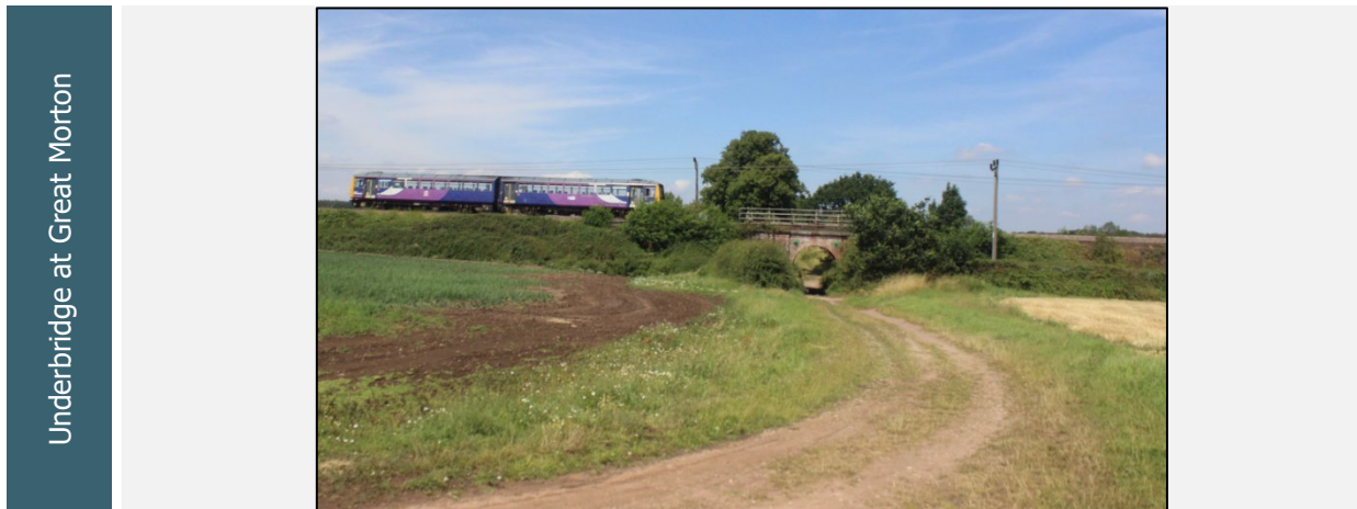
Figure 4: Underbridge at Great Morton
