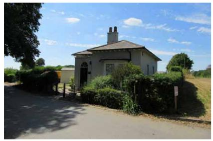
Fig 204: Bishopfield Lodge is an endearing mid-19th century lodge building. It has a rendered, single-storey form and a hipped natural slate roof with timber bracketed eaves and a tall chimney stack. Its fenestration includes a canted bay window bay and timber '2 over 2' sashes.
