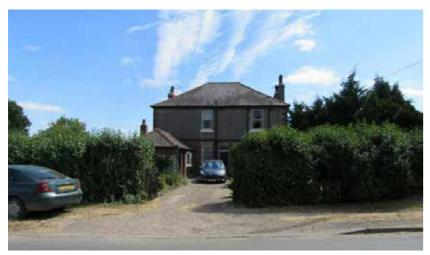
Fig 205: The two-storey farmhouse opposite Scrooby Top House has a classic interwar aesthetic, with differing in external finishes between ground and first floor levels (exposed red brick with pebbledash render above), and hipped slate roof with clay ridge tiles and red brick chimney stacks.
