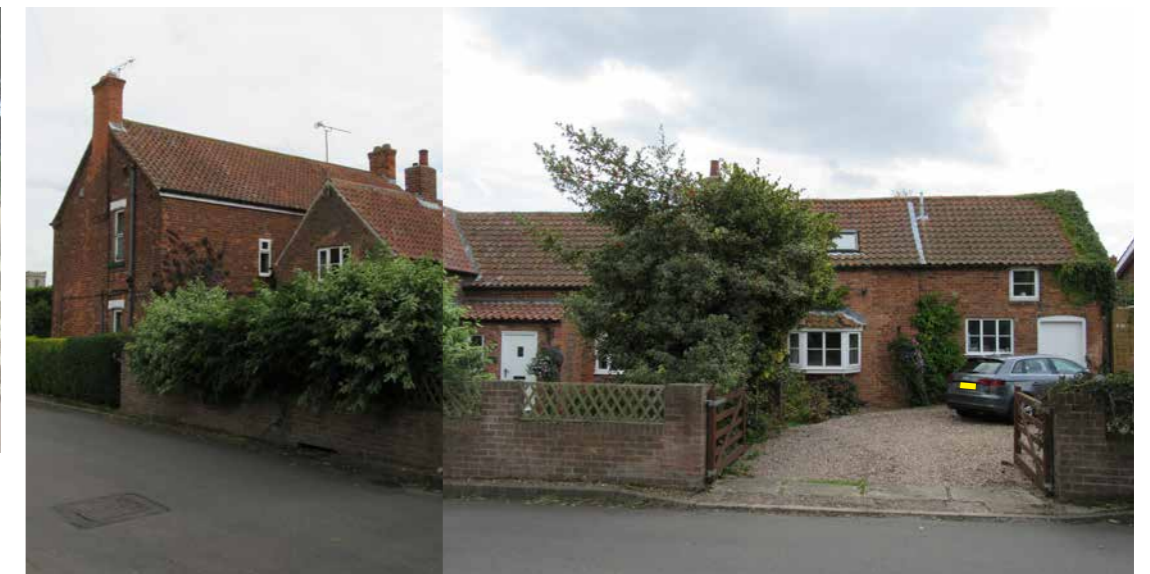
Fig 195: The 18th century Holly Cottage, which also includes some 19th century additions, is an attractive residence built in the local vernacular style. Its red brick form features Flemish bond brickwork and dentilated eaves. Chimney stacks emerge from along the ridge of its pitched clay pantile roof.
