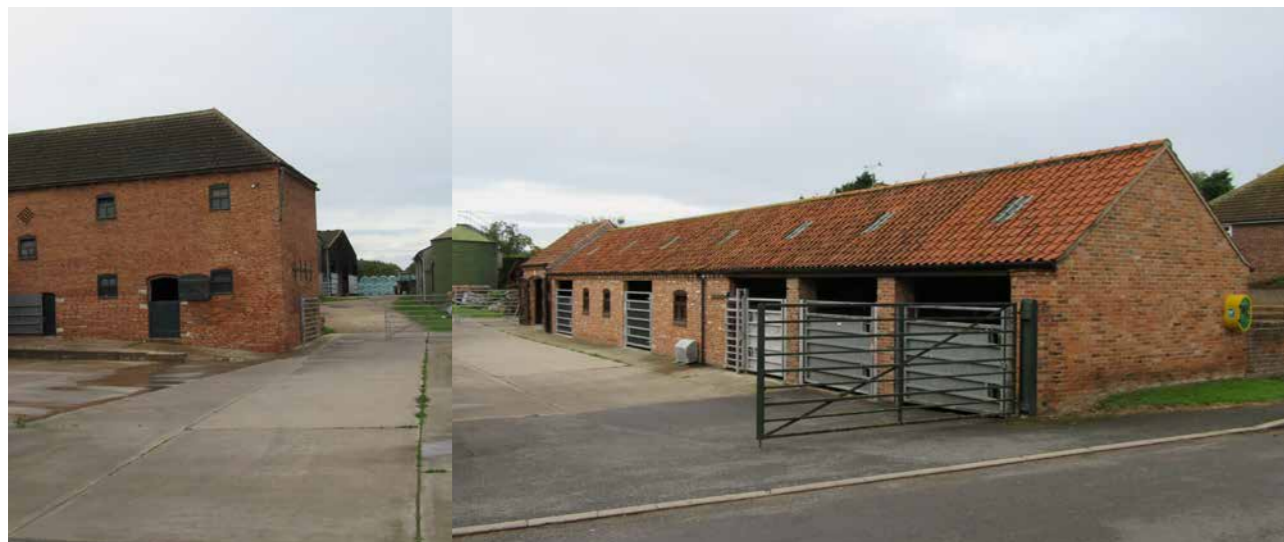
Fig 193: Of similar design and aesthetic to Rampton's other vernacular farm clusters, the late-18th/early-19th century buildings to Home Farm include a large two storey threshing barn and single storey stables, animal sheds and store. The threshing barn features some particularly pleasing details, including stone dressings, diamond pattern ventilators, and full height openings with timber doors.
