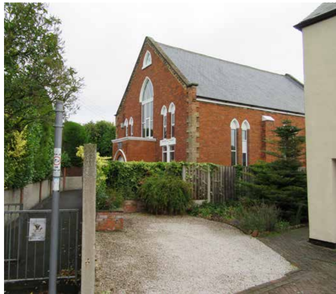
Fig 183 and 184: A private residence since its closure in 1992, the old Methodist Chapel buildings are set back from Main Street. Built in 1857, the chapel is one of Rampton's most distinct and eye-catching buildings. It has an elegant red brick form with slate roof, with symmetrical façade framed by buff brick quoins and hosting a central porch with gothic arched opening.
