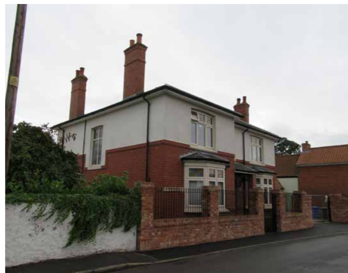
Fig 197: Originally a public house and guest house, Royal Oak House still possesses the air of a landmark building despite having been converted to a residence in more recent years. It has an appealing aesthetic, defined by its half-red brick, half rendered facade treatment, ground floor bay windows, and shallow slate hipped roof with tall chimney stacks.
