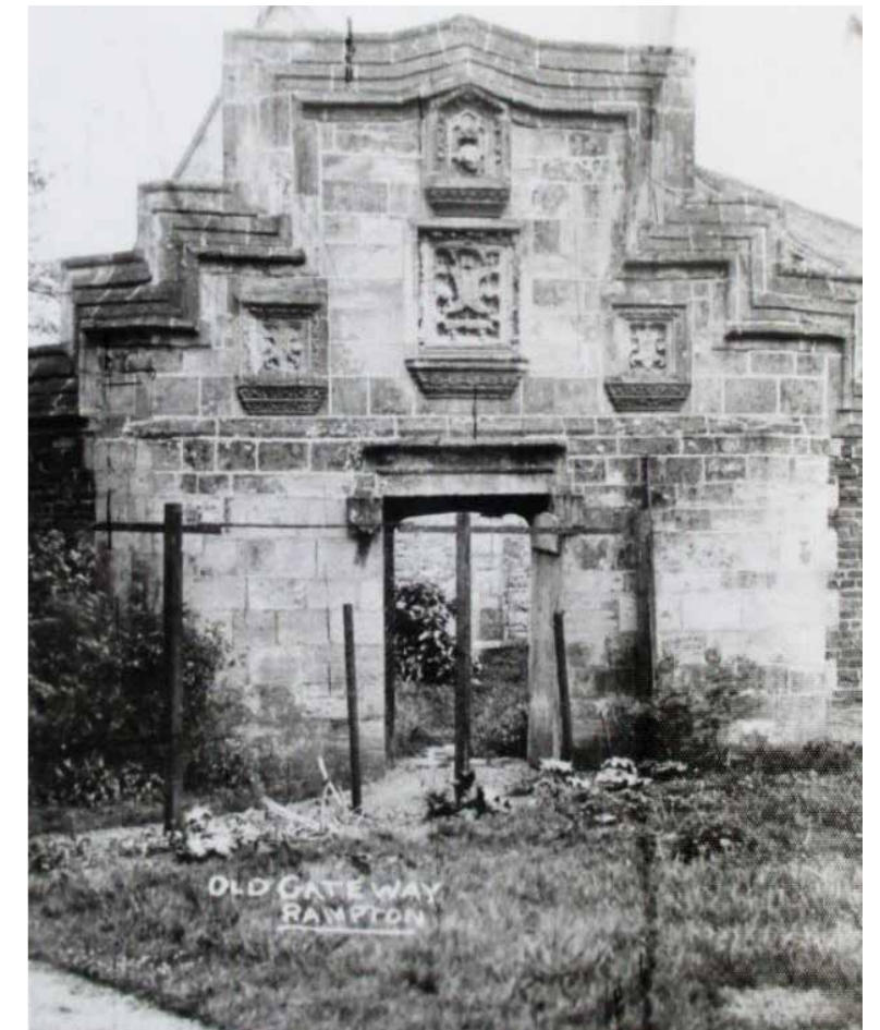
Fig 59: Described by Pevsner as “an uncommonly lavish piece of Early Tudor brickwork, rising in three stepped stages and adorned with corbelled-out panels of terracotta with coats of arms”, the early 16th century gateway is the only lasting remnant of the original Manor House.
