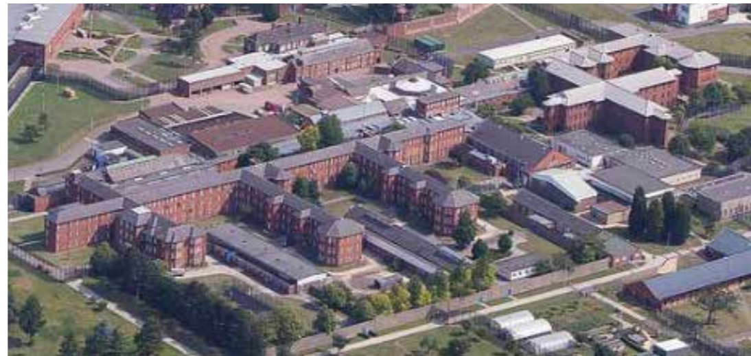
Fig 271: Positioned within a secured setting and largely screened in views from the more accessible parts of the hospital grounds, are the original buildings of Rampton Criminal Lunatic Asylum. Designed by Francis William Troup and constructed in the early 1910's, the hospital complex is built of red brick with natural slate roofs. It is formed of a main west-to-east wing, 4 interconnecting cross-wings, which meet the main wing at 90° angles along its length, resulting a grid layout with a series of enclosed and overlooked central spaces.
