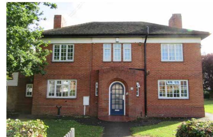
Fig 277: The former Chaplain's house on Galen Avenue dates from 1929. A red brick, two-storey dwelling with hipped rosemary tile roof, the property has a symmetrical façade with a central recessed brick door opening, the design of which echoes that of the entrance to the administrative block, albeit in a much more modest and domestic scale.
