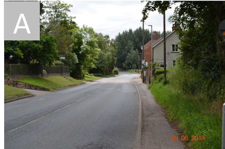
View looking towards Blyth Village. Bus Stop outside grey house on left (Shincliffe House). Houses on right are set back from the road.
