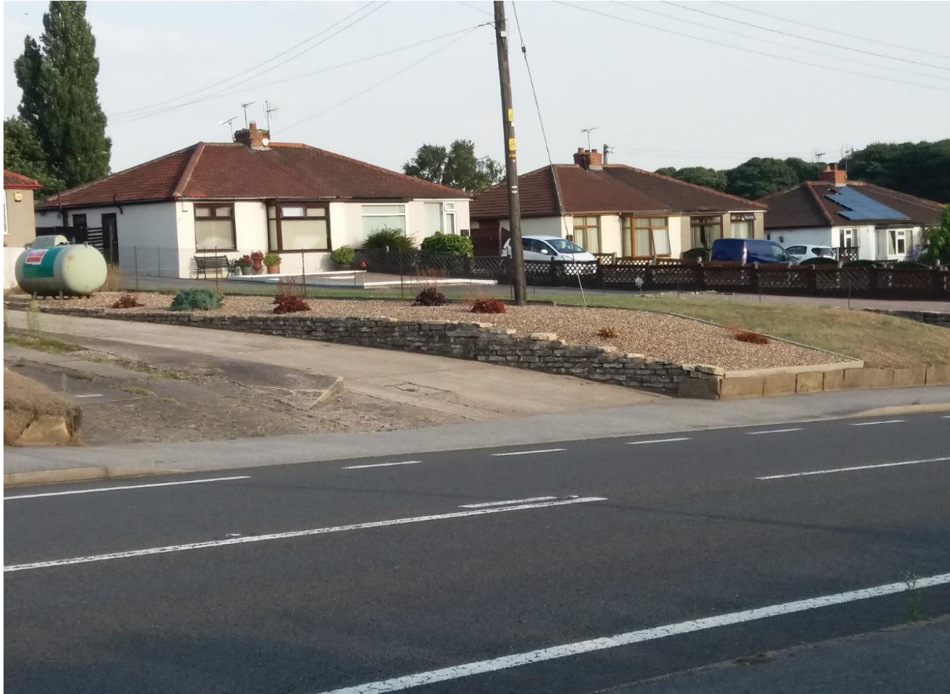
Typical semi-detached Bungalows, Bawtry
