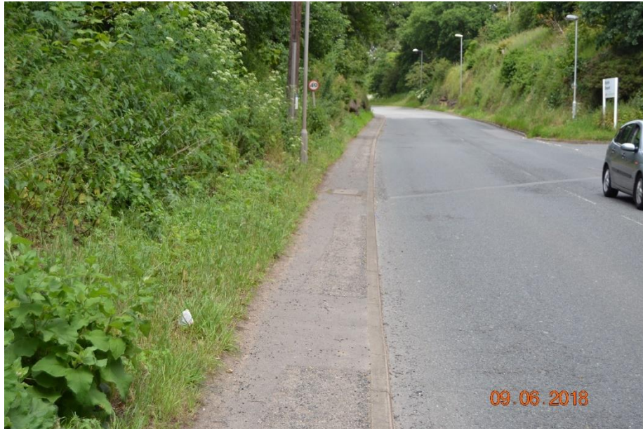
Bawtry Road. Note very narrow pavement, not wide enough for wheelchairs, prams etc., and dangerous for pedestrians because of speeding lorries coming up behind them.
