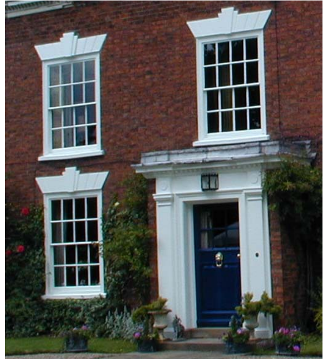
18th Century Sash windows in Rushcliffe make a significant contribution to this fine building.
