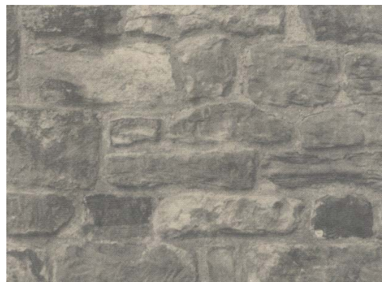
Good repointing of stonework.
