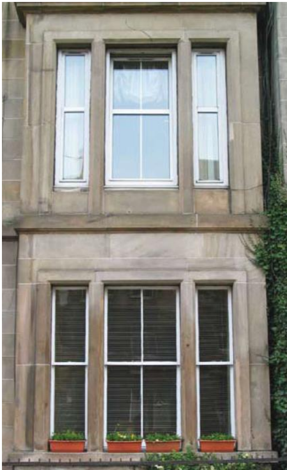
The top window has been replaced with uPVC windows whilst the bottom retains the original timber frame and glass. The replacement of the traditional sash changes the character and appearance of the building and has an overall detrimental effect on the aesthetics of the façade.
