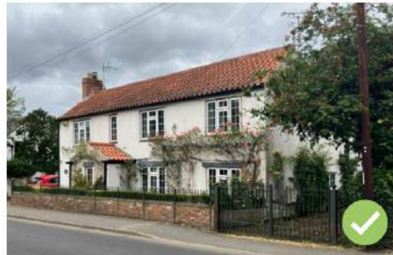
Figure 17: Variation in setback allows for a variety of on-plot parking solutions. Here, a side-driveway provides access to a garage at the rear of the plot, ensuring frontages are not dominated by parking.
