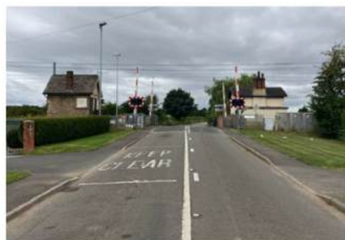
Figure 43: The level crossing on Station Road creates a defined entry point or 'gateway' to the village.
