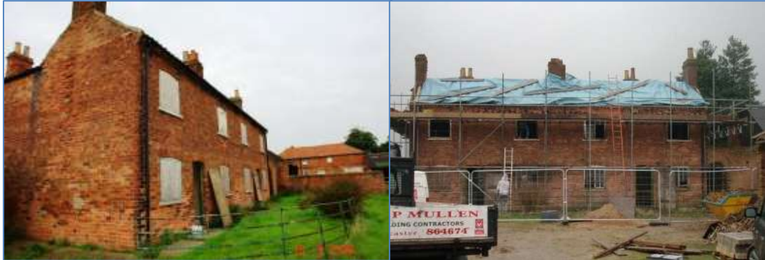
The cottages before and during repairs
