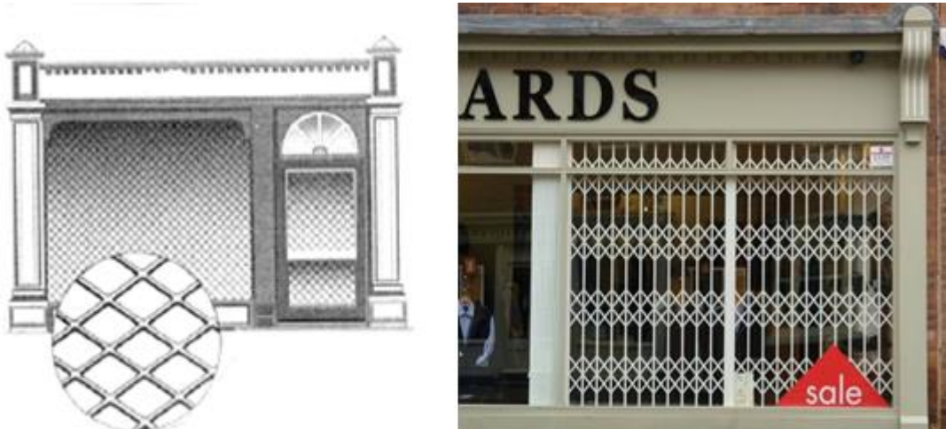
Figure 58. Examples of internal grilles (drawing courtesy of Rutland County Council).
