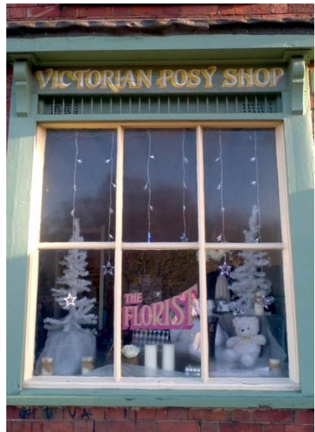
Figure 53. Small panes of glass are easier and more cost effective to replace if smashed.
