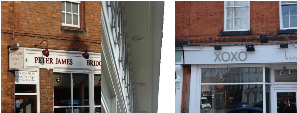
Figure 46. Left; swan neck lights. Middle; spotlights discretely set in a modern cornice. Right; unsightly oversized spotlights to illuminate fascia.
