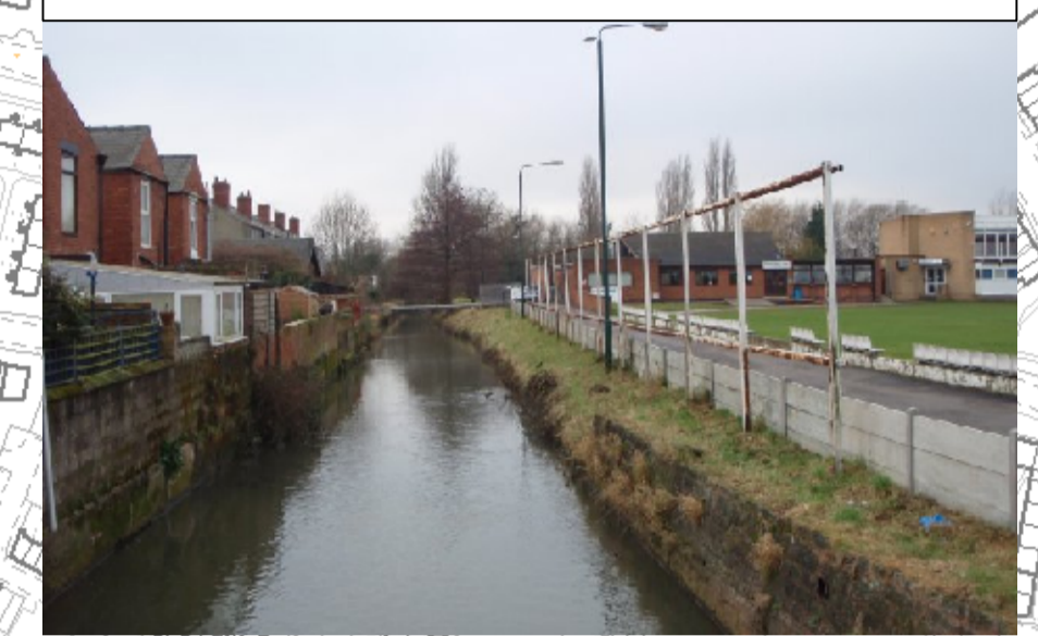
Left bank height sufficient to contain a 1 in 20 annual chance flood. Informal cricket pitch boundary wall cannot be relied upon to contain 1 in 100 annual chance event.
