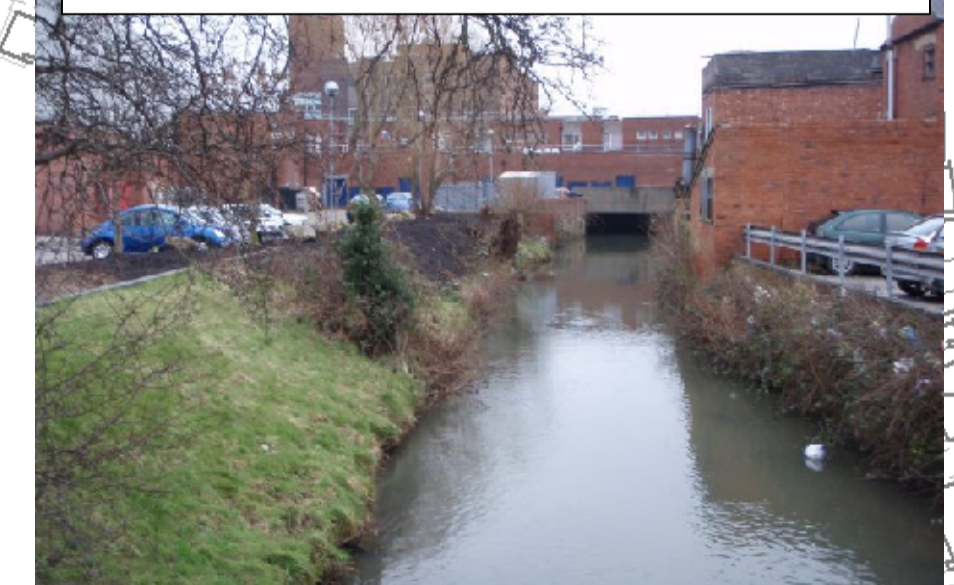
Looking downstream with EA maintained left bank defence
