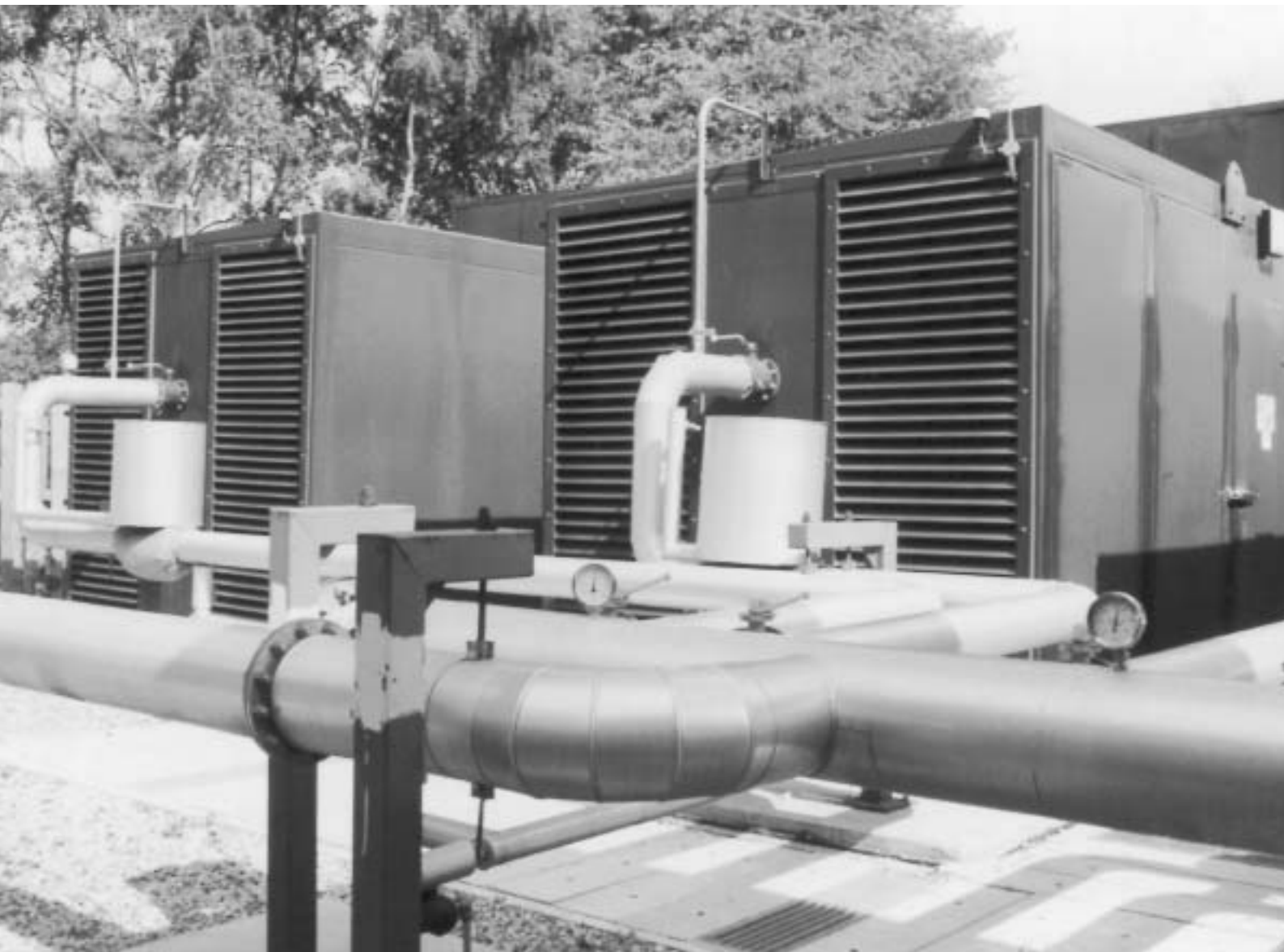
Electricity generators at Burntstump Landfill Site, Calverton. This is one of 5 landfill sites in the County where landfill gas is collected and burnt to generate electricity.
