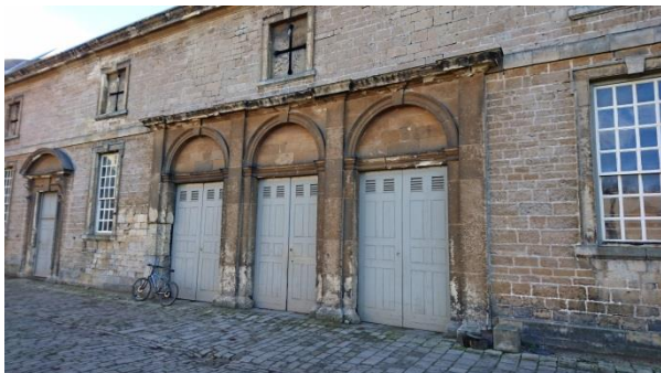
West elevation of c1704 range, east block, north section (courtyard face) – note the first floor crucifix vents.
