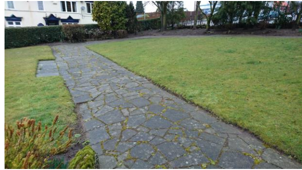
Crazy-paving (of broken concrete slabs) in 1960s extension.
