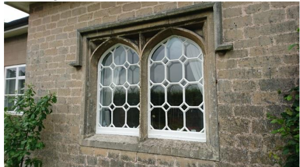
Gothic windows and hood moulds at East Lodge.
