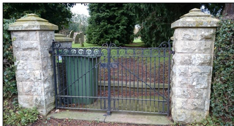
Gate piers and gates at main entrance
