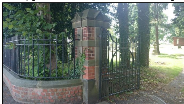
Front boundary wall, railings, gate piers and gates
