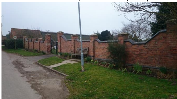
Front boundary wall
