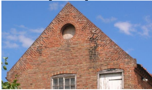
Figure 6.39: Example of 'tumbling in' on an agricultural building in Hayton.
