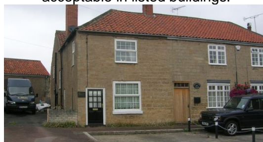
Figure 6.49: The installation of UPVC windows has caused harm to this significant building within the Carlton in Lindrick Conservation Area.
