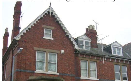
Figure 6.43: Decorative timber bargeboards and fascias with brackets, common features of late-19 th century villas (particularly in Worksop and Retford).
