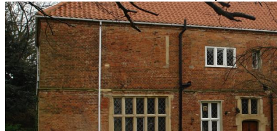
Figure 6.63: large in-filled window opening on a c1600 building in Walkeringham.
