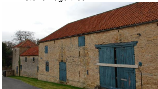
Figure 6.30: A traditional pantile roof from the late-18 th century.
