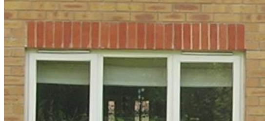
Figure 6.21: Vertical soldier arch – This is not normally suitable on historic buildings.
