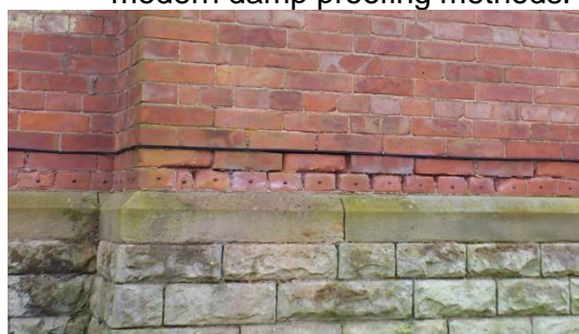
Figure 6.83: A damp proof course has had a noticeable impact on the appearance of this building within the Oldcotes Conservation Area.
