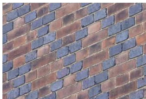
Figure 6.3: An example of diaper brickwork.
