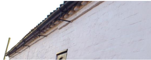
Figure 6.45: Hal-round cast iron guttering on rise and fall brackets.
