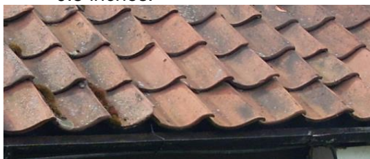
Figure 6.29: Typical pantile roof.
