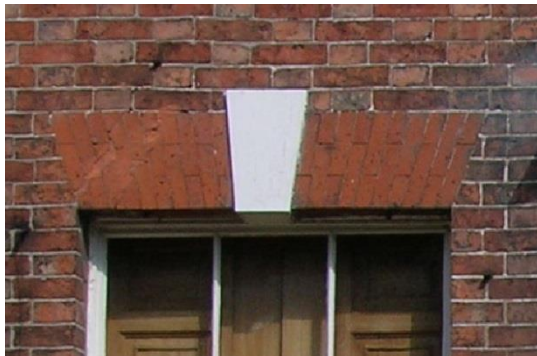
Figure 6.16: Flat head arch of rubbed brick with voussoir/keystone.
