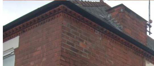
Figure 6.42: Distinctive eaves detailing of late-19 th /early-20 th century terraces in Worksop, with rows of terracotta tiles of various patterns.
