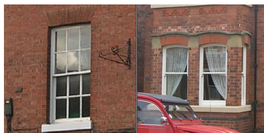
Figure 6.51: Comparison between 18 th century '6 over 6' sash window with its small panes and squared meeting rail (left) and a late-19 th century '1 over 1' sash with larger panes and horns at the meeting rail (right).
