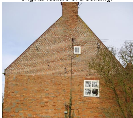
Figure 6.38: Raised gables and decorative 'tumbling in' at the verges.
