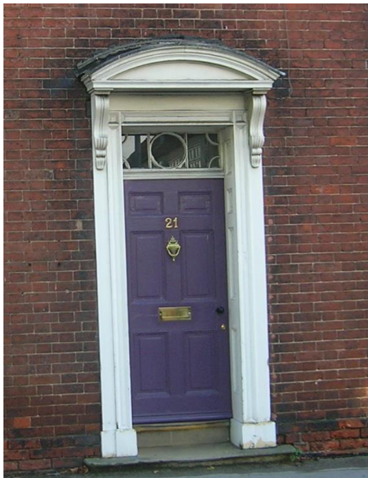
Figure 6.68: A typical Georgian 6-panel door with door case and fanlight.
