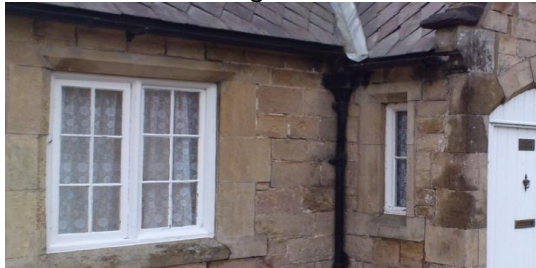
Figure 6.60: Timber mullion window in a mid-19 th century lodge in Oldcotes.
