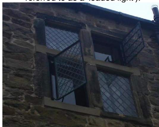
Figure 6.55: Stone cross-casement window with iron-framed leaded casements.
