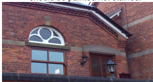
Figure 6.81: The stained joinery in this converted coach house in the Oldcotes Conservation Area is at odds with the original painted joinery and is inappropriate in this historic setting.
