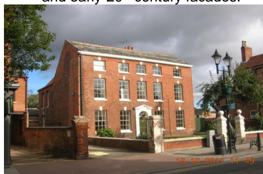
Figure 6.50: Mid-18 th century vertical sliding sashes ('6 over 6') in grade II* listed building on Grove Street, Retford.
