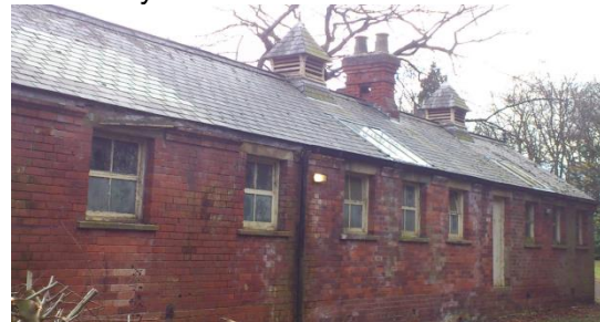
Figure 6.58: Hopper-style windows in a former kennels building at Oldcotes.
