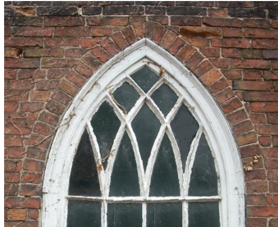
Figure 6.19: Gothic-style arch.
