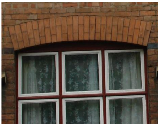
Figure 6.18: Cambered arch of rubbed brick.
