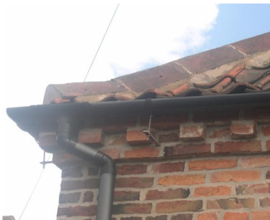
Figure 6.41: Example of dentil course with projecting header bricks.
