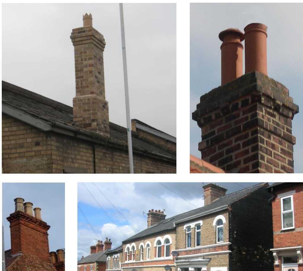
Figure 6.2: Traditionally detailed chimneys with pots add much character to the skyline. Chimneys often include sawtooth brickwork or oversailing courses. Sympathetic repairs and/or replacements (such as the rebuilt chimney at Worksop Railway Station, top left) also help preserve the significance of heritage assets.
