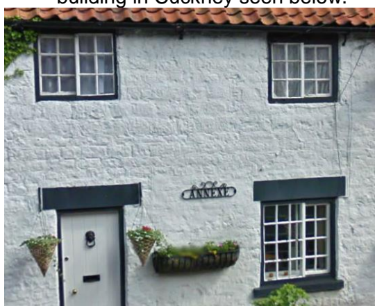
Figure 6.54: '12 by 12' and '6 by 6' horizontal sliding sashes at Cuckney.
