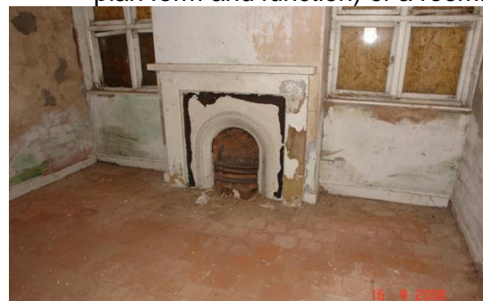
Figure 6.89: Chimney breast, surround and insert with hob grate all add much to the appearance and form of this 18 th century listed building in Mattersey.
