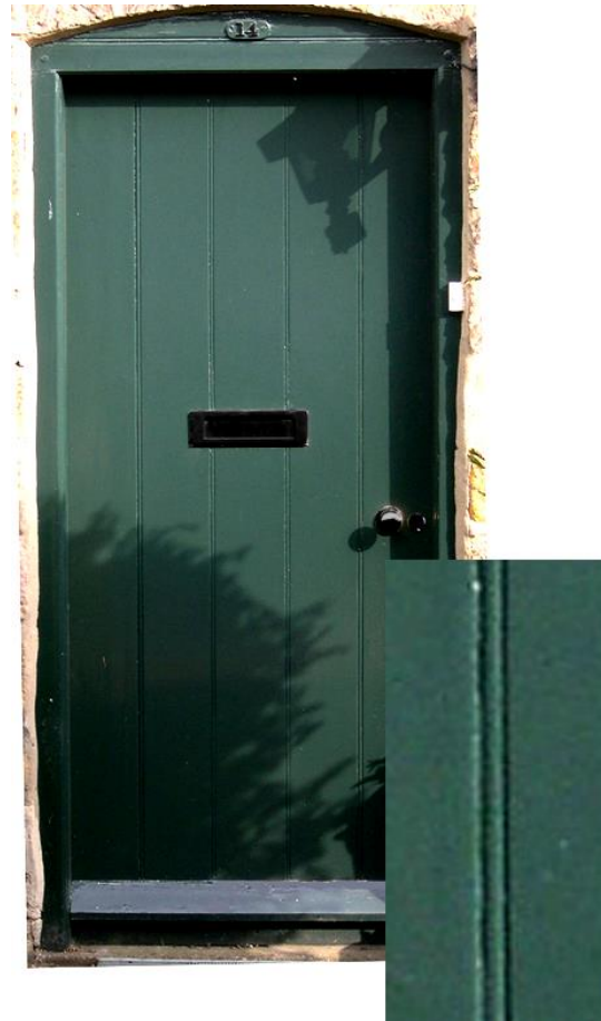
Figure 6.67: A simple plank door with scratch moulding.
