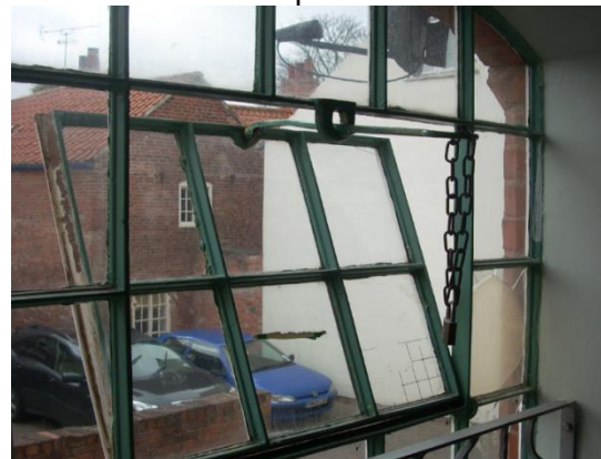
Figure 6.59: A hopper-style metal-framed window, complete with stay, in a mid-19 th century industrial building off Bridge Street, Worksop.
