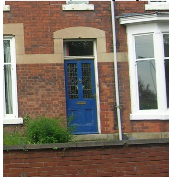
Figure 6.69: Typical 4-panel Victorian door with glazed and leaded upper panels on Blyth Road, Worksop.
