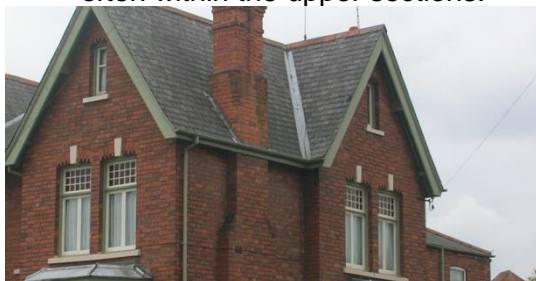
Figure 6.61: Transom window with flush-fitting side-opening casements below and coloured non-opening lights above, in a c1895 villa in Worksop.
