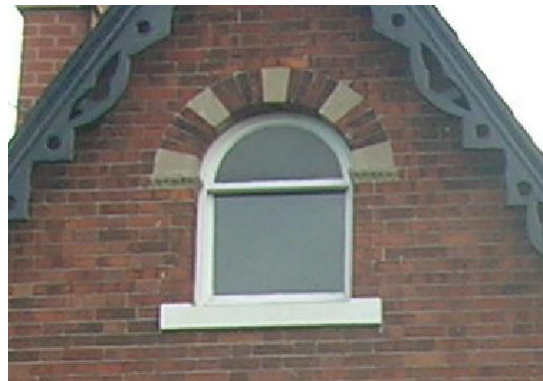
Figure 6.20: Round-headed arch.
