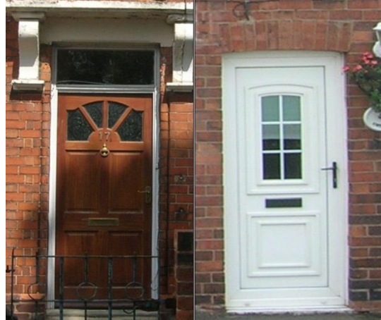
Figure 6.79: Left: A modern door with integral fanlight in stained finish. This style of door and finish is unsuitable in listed buildings and in Conservation Areas; Right: A modern UPVC door is never acceptable in listed buildings or Conservation Areas.
