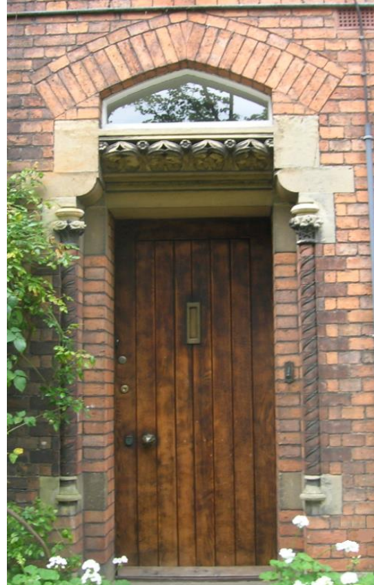
Figure 6.73: Mid-Victorian doorway in Retford, in the Gothic revival style – with intricately carved foliated detailing and pointed brick arch.
