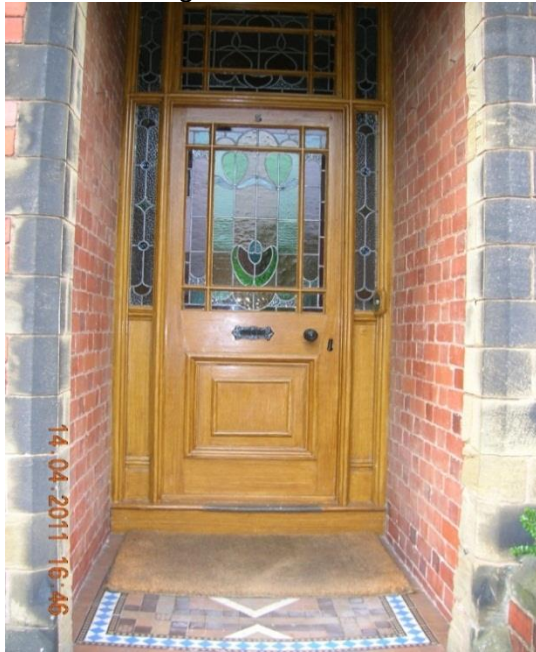
Figure 6.71: Late-19 th century two-panel door on Blyth Grove, Worksop, with leaded glazing panels containing coloured glass. Also note the margin sidelights and overlight.
