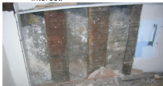
Figure 6.86: 16 th century timber framing (previously hidden behind the plaster) in this listed building in Worksop.
