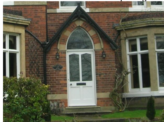
Figure 6.70: Gothic arched opening with pointed fanlight and shallow-pointed glazed door panels on this mid-19 th century villa in Worksop.
