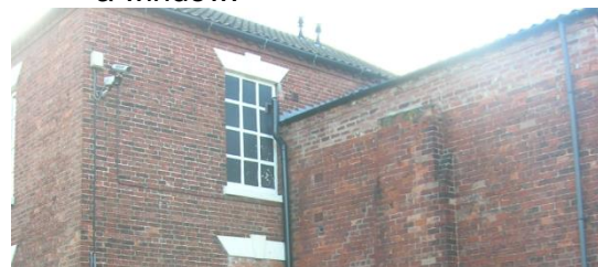
Figure 6.64: Tax-relief opening with painted detail on a c1800 former Vicarage in Worksop.
