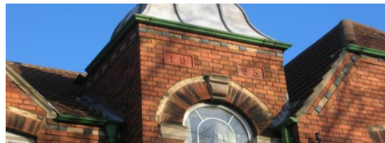
Figure 6.46: Ogee-style cast iron guttering on late-19 th century villa in Retford.
