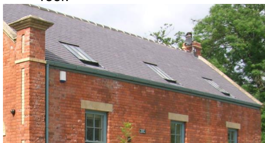
Figure 6.37: Flush-fitting conservation style rooflights in Shireoaks Conservation Area.
