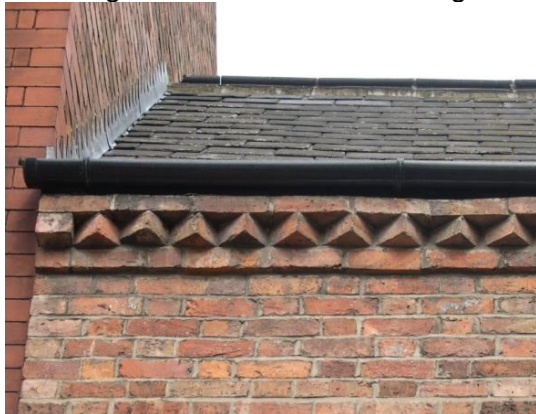
Figure 6.40: Example of 'Sawtooth' brickwork.
