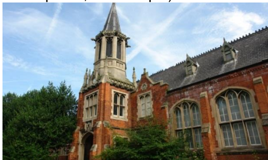
Figure 6.22: Stone is used here for quoins, mullions, tracery, copings and bell tower.
