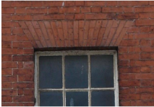
Figure 6.15: Flat head arch of rubbed brick.
