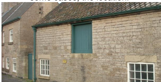
Figure 6.82: Painted joinery and rainwater goods in cream and blue/green estate colours, in this listed building within Holbeck Conservation Area.
