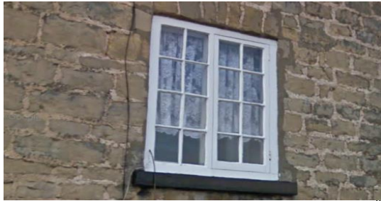
Figure 6.57: Traditional flush-fitting late-18 th century casement window at Cuckney.
